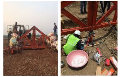
Plate Load Test (Warangal)
