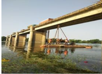
Under water drilling (Bheema River)
