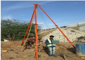
Rotary drilling (Tamilnadu)
