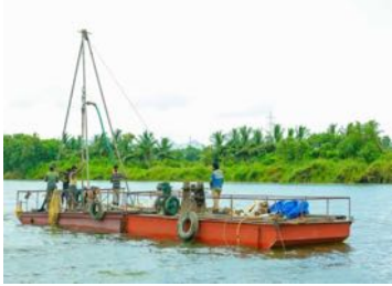
Under water drilling (Krishna River)
